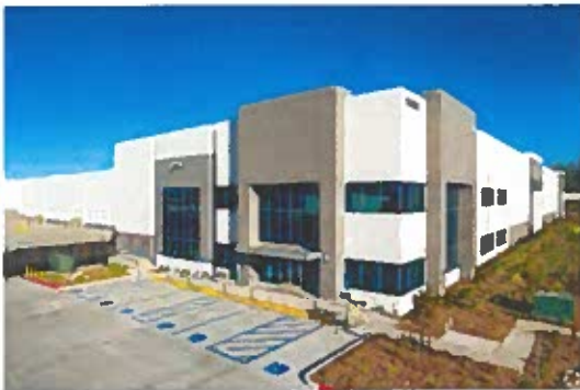
Typical Building Design with Concrete Wall Panels
