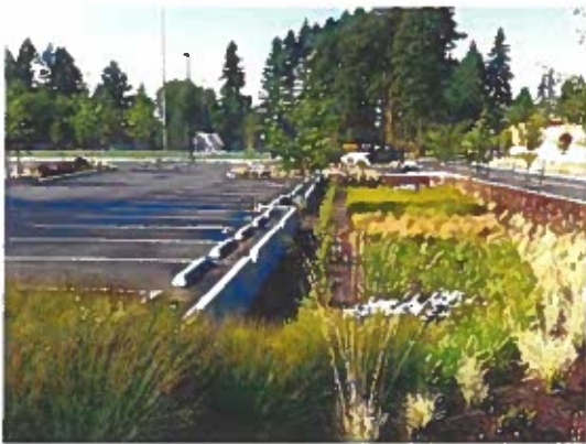
Vegetated Bioswales are Encouraged in Parking Lots
