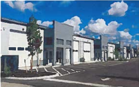
Typical Industrial Flcx
